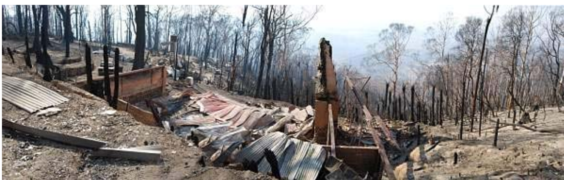
Figure 8 Destroyed timber house at the bottom (south) of Pine Ridge Road: looking south toward Strathewen, the Mount Sugarloaf ridge is at the right (west) [note the close proximity of trees].
