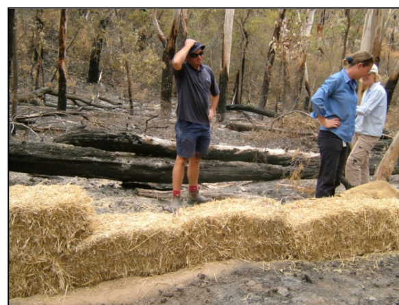
Figure 3: Installing sediment barrier traps
